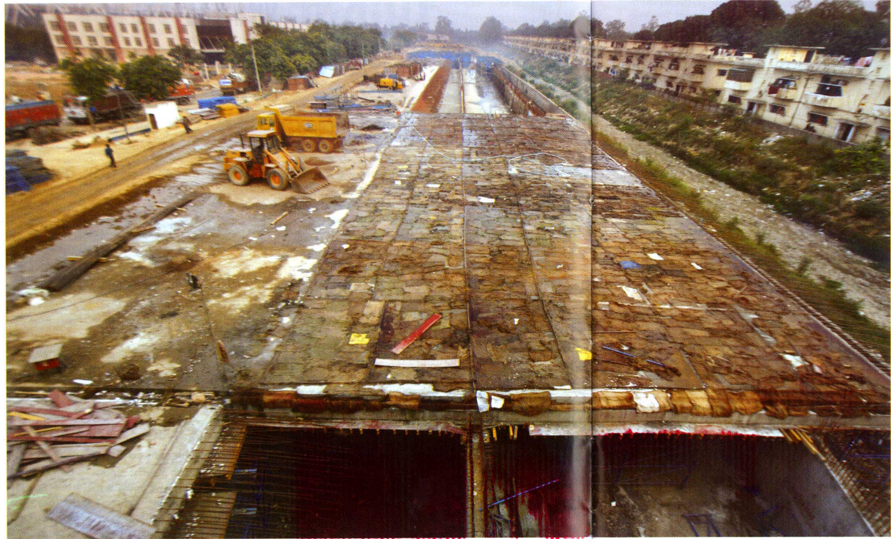
Stretch of a nullah being covered up to make a parking lot for the Commonwealth Games
